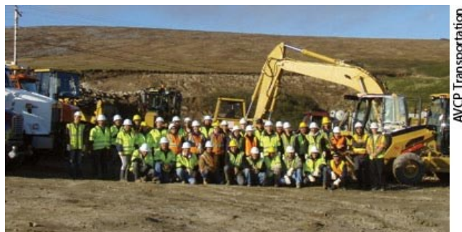
These force account workers representing the Association of Village Council Presidents pose in front of the equipment they are using to construct a project on tribal land.
